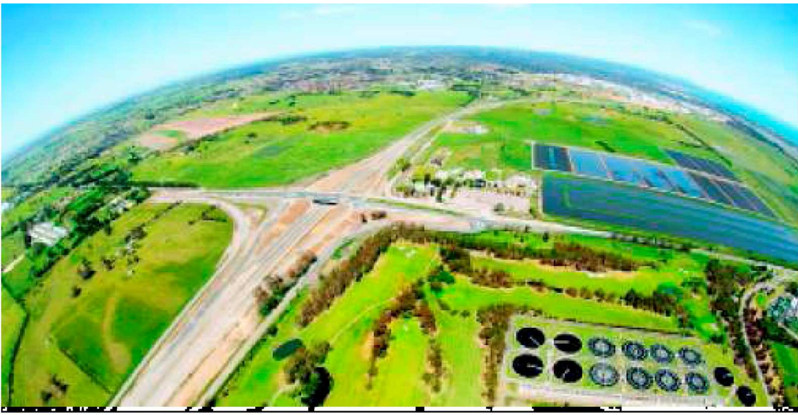
The EastLink takes shape at Thompsons Rd, Carrum Downs.
