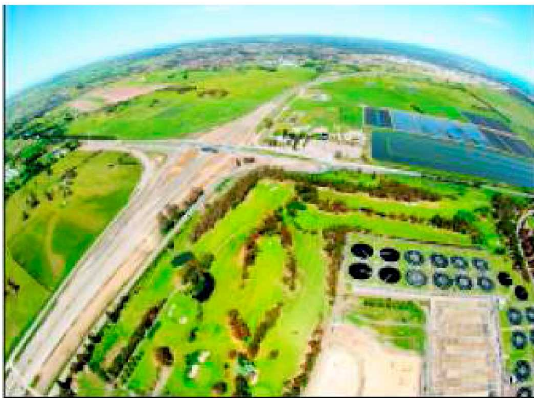
The first stage of the $42 million EastLink Business Park in Carrum Downs has nearly sold out.
